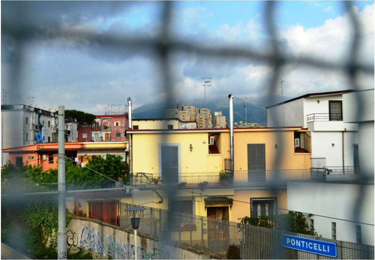
PHOTO 7: View of the Circumvesuviana station at Ponticelli from the overpass, May 2018
