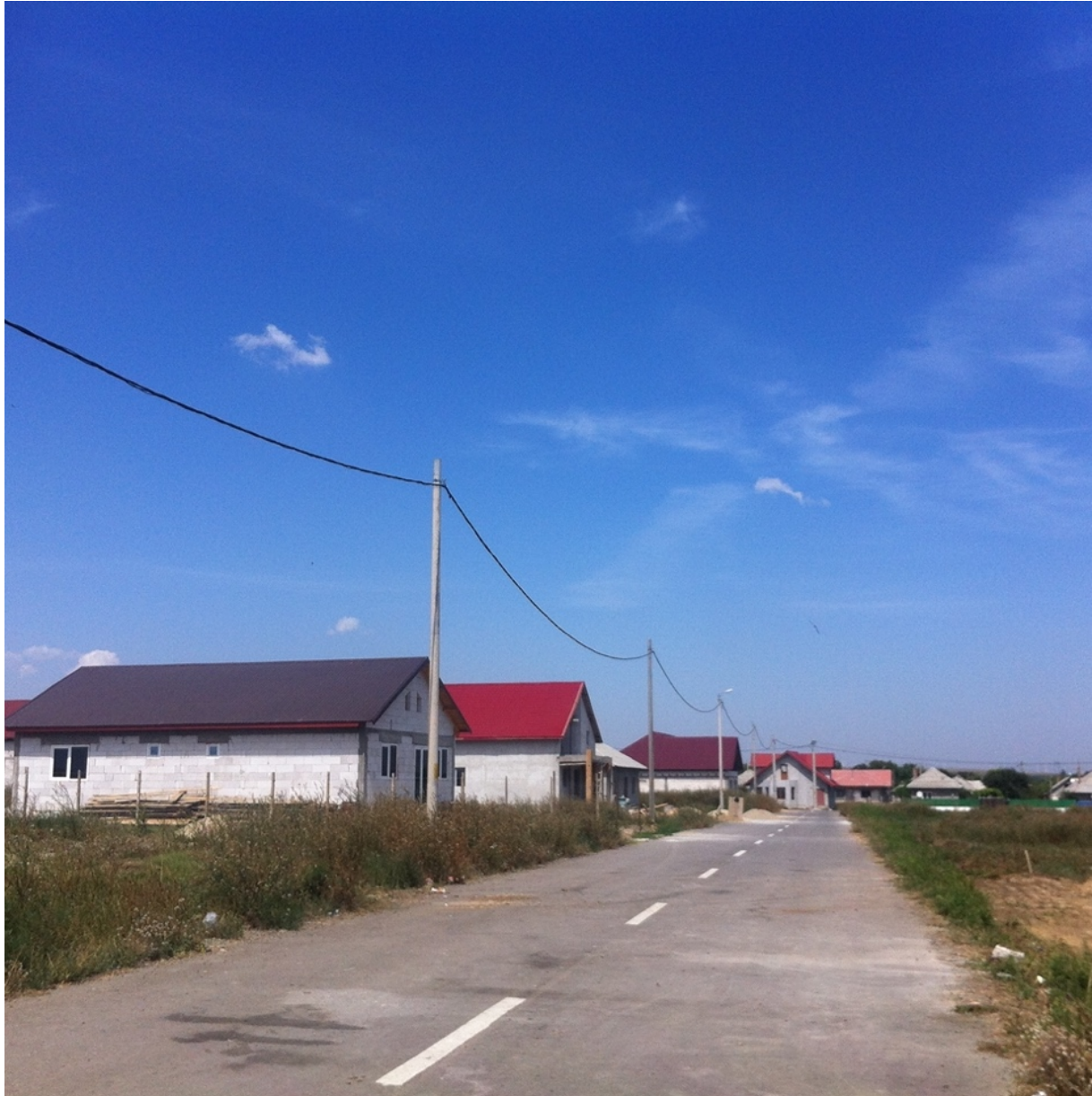
FIGURE 10: Road in the new part of Sibiu Mare, 2015
