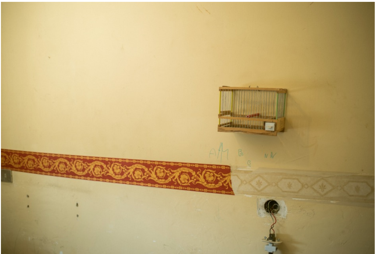
PHOTO 20: Wall of a room
