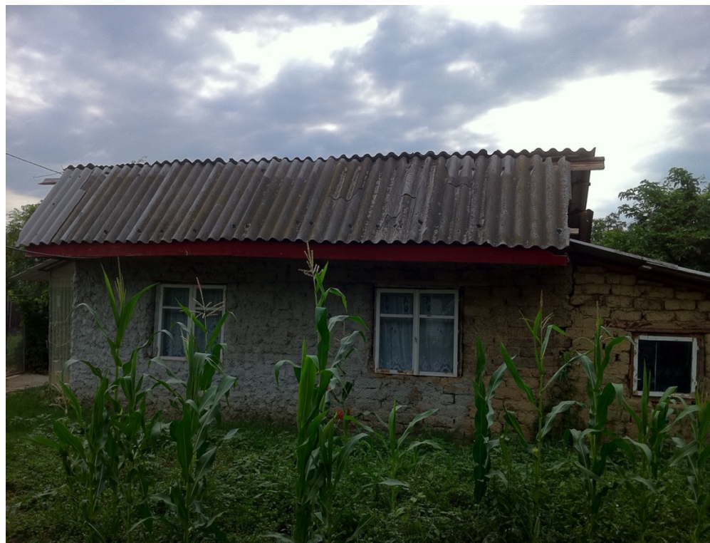
FIGURE 22: House in adobe with the roof redone in metal sheets before the migration
