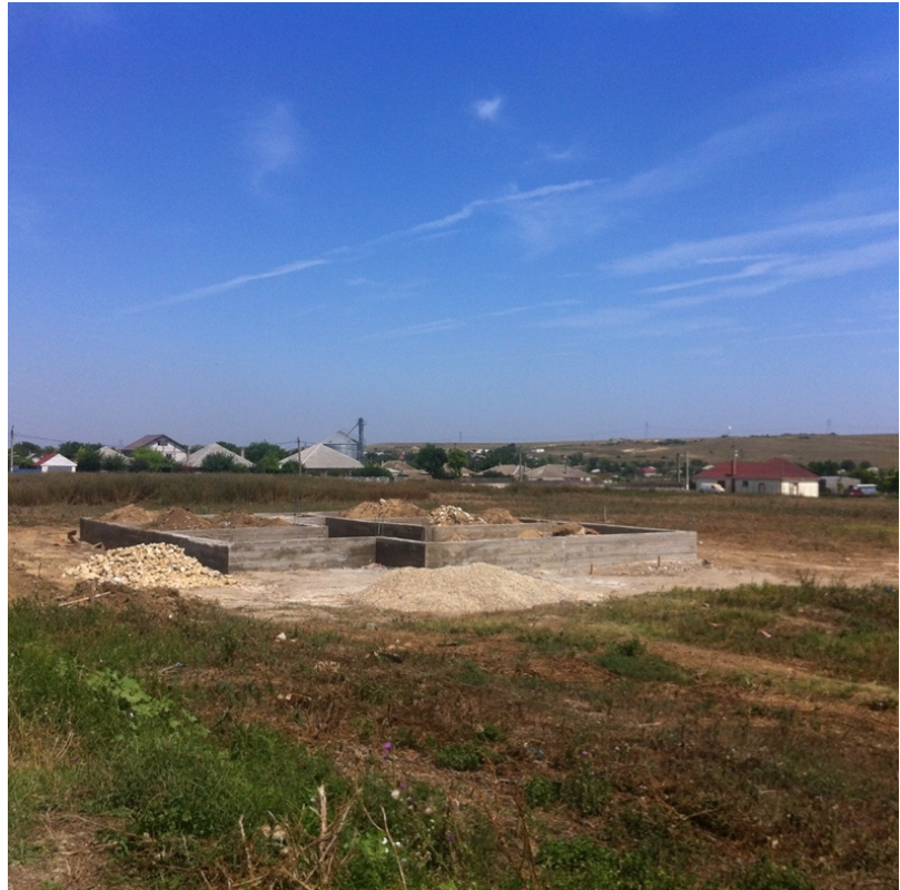
FIGURE 25: Foundations in the new part
