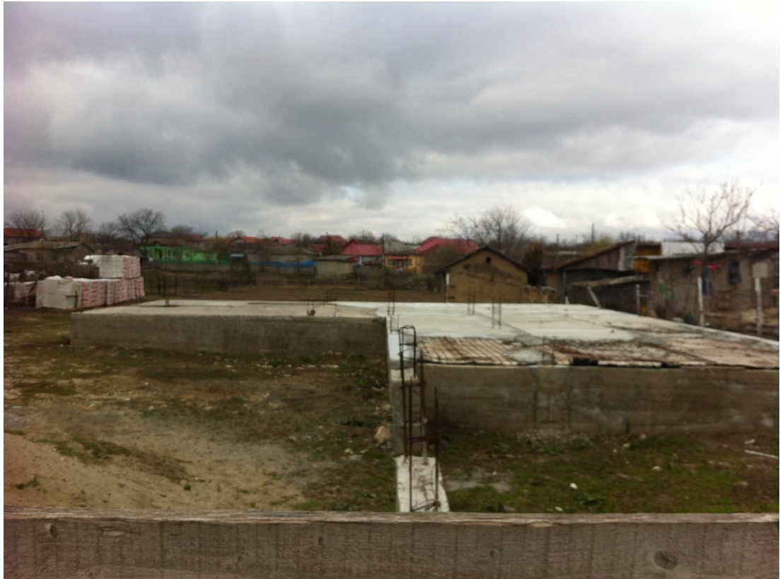
FIGURE 23: Foundations in the new part of the village defined 'case vechi'
