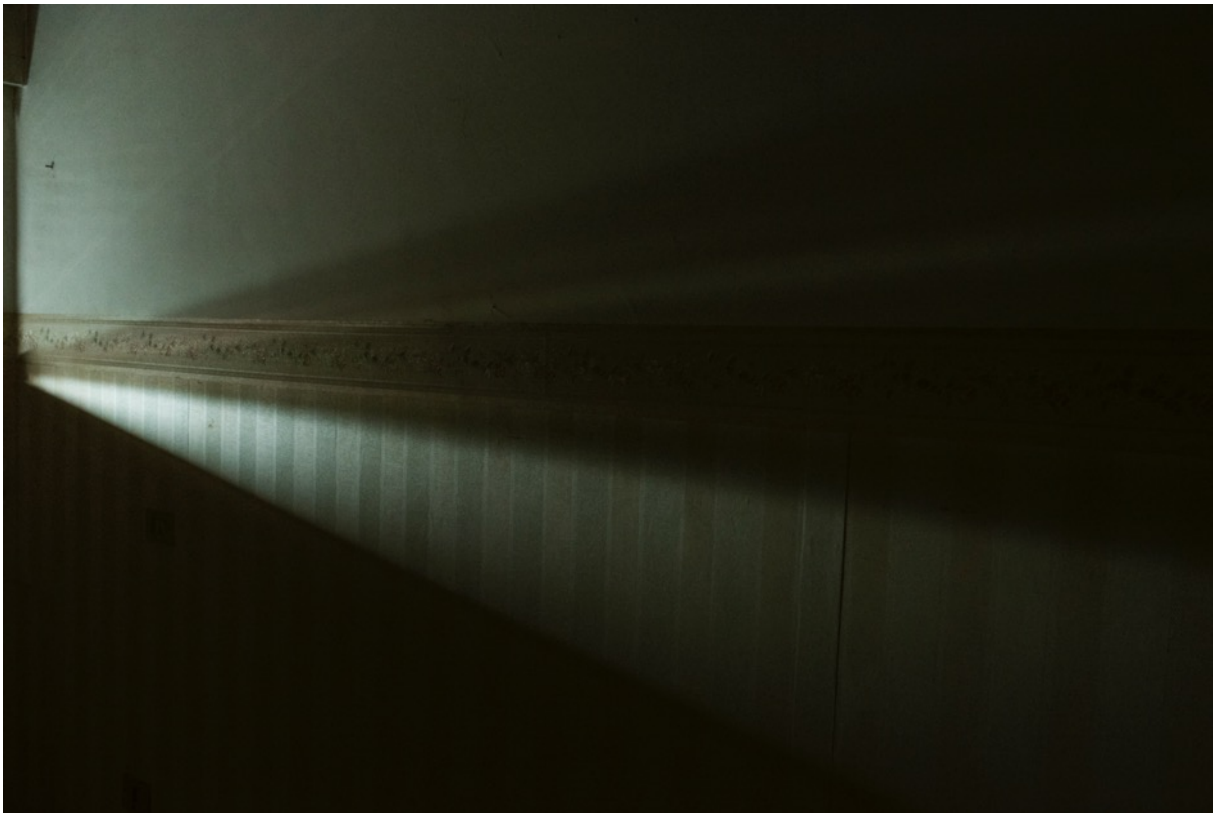
PHOTO 86: Detail of the wall of one of the motel rooms
