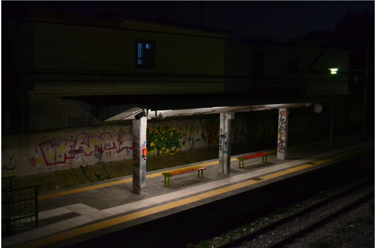
PHOTO 21: The Circumvesuviana station at Ponticelli, platform, February 2019
