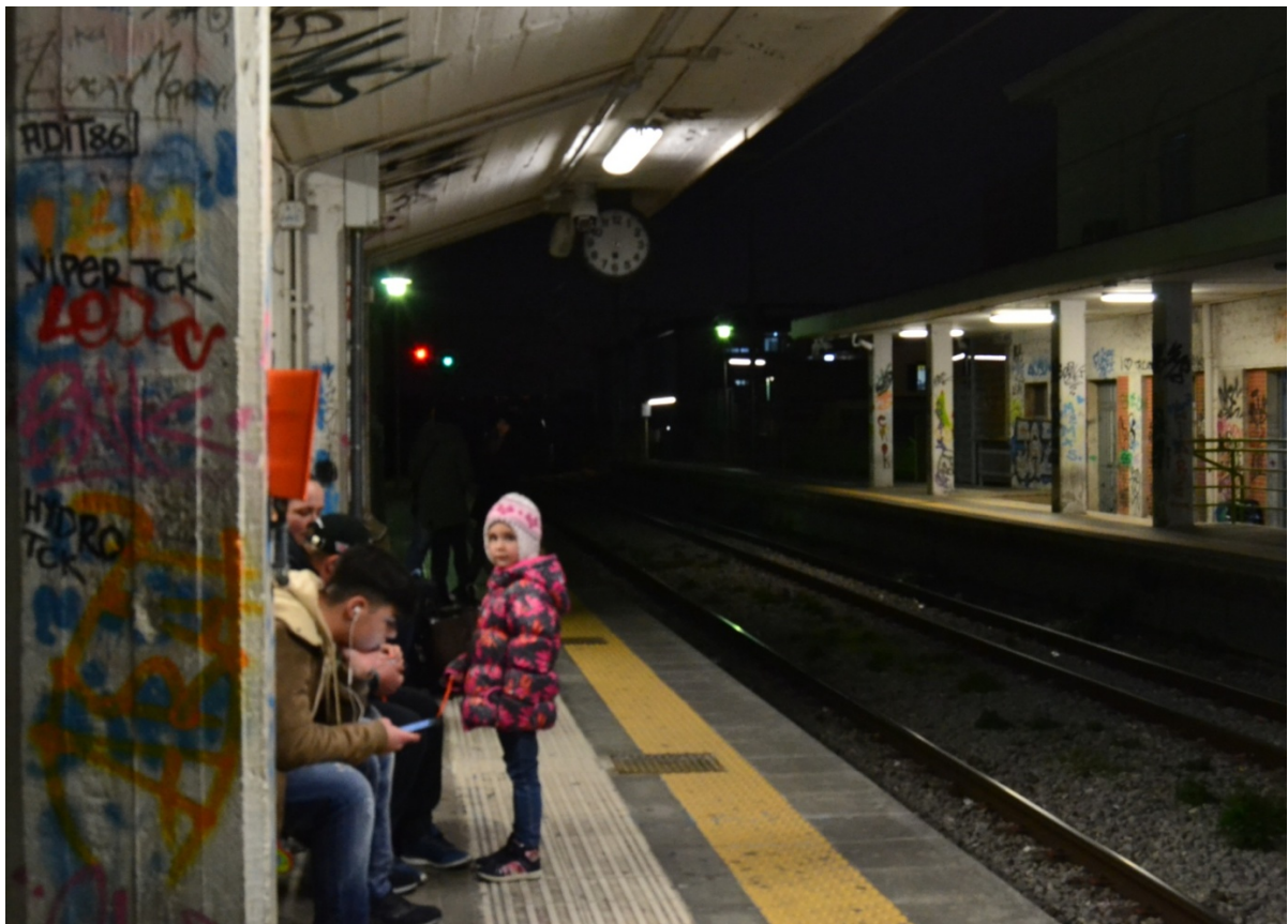
PHOTO 20: The Circumvesuviana station at Ponticelli, passengers waiting, February 2019
