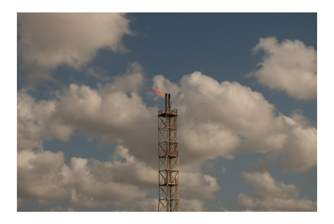
**PHOTO 18:** Gela, refinery. Torch chimney in operation. The torches burn the gases eliminated in the production plant.
