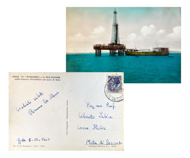
**PHOTO 10:** The first offshore drilling rig in Europe (1958), built in the United States and called "Scarabeo", together with the Saipem motor ship, used for oil exploration at sea. Postcard.
