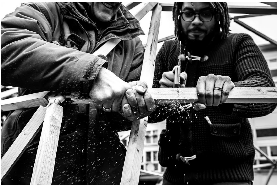
PHOTO 10: Construction of the geodesic orchard.
